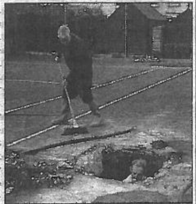
• Tom Murphy and Pat Hanley hard at work in preparation for the new lighting. (P).
